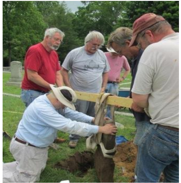
Above: lifting out a leaner to reset it nice and straight.
